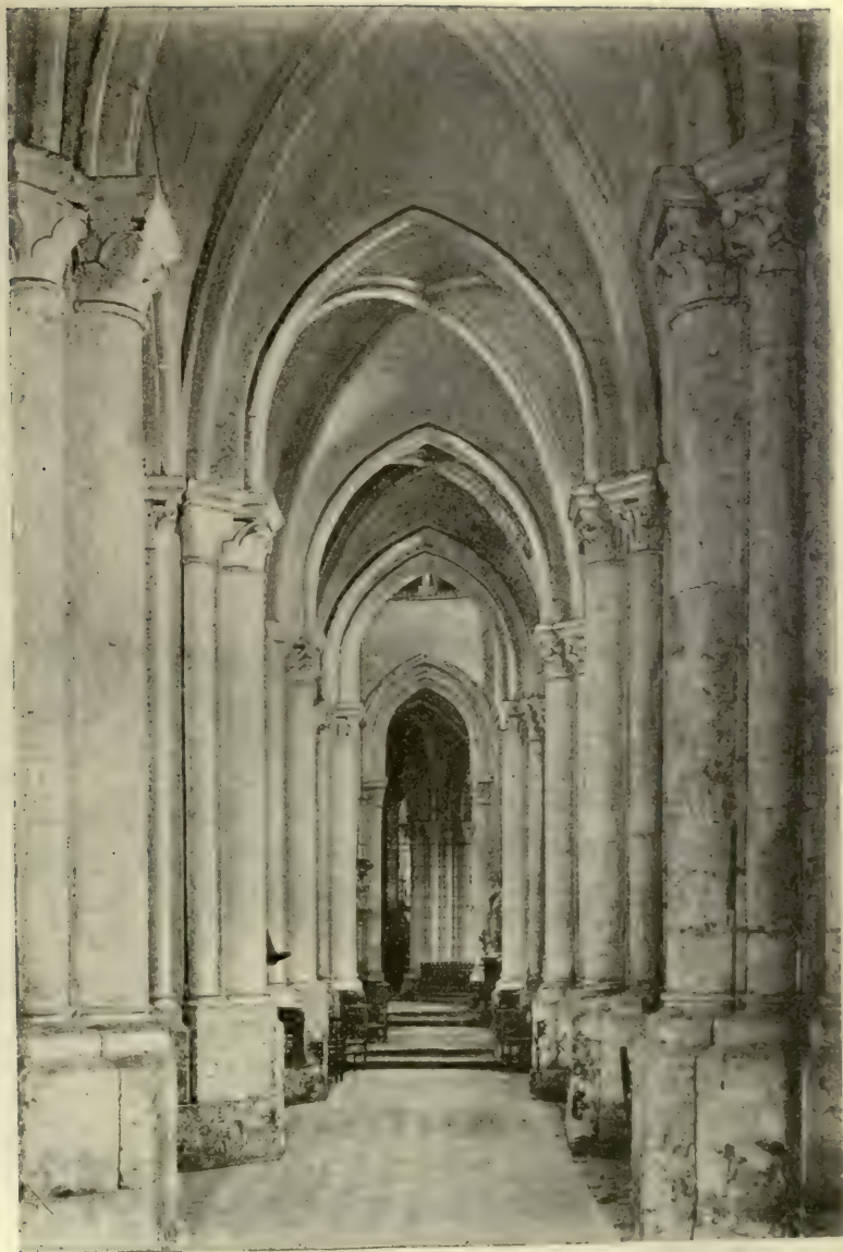
SOUTH AISLE, LOOKING EAST Abbey Church, St. Germer
